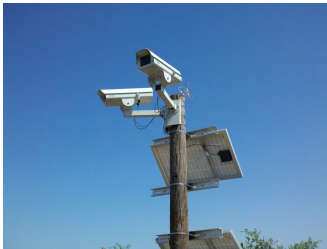
One or more cameras on AC or Solar Power
